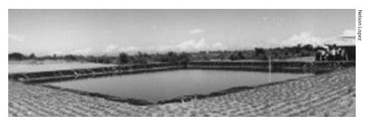
**Photo #9. A fish pond** located in a coastal wasteland. Special plastic lining (for example made of polyethylene) is used as ground cover which functions as a hydraulic barrier to pond dikes and bottoms. The pond liner is used for water containment and helps preserve biosecurity by preventing pathogens from entering and infecting the pond.
